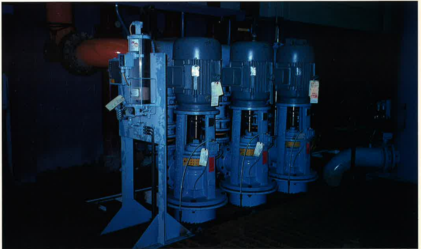
Three vertical turbine pumps on central coolant service.
